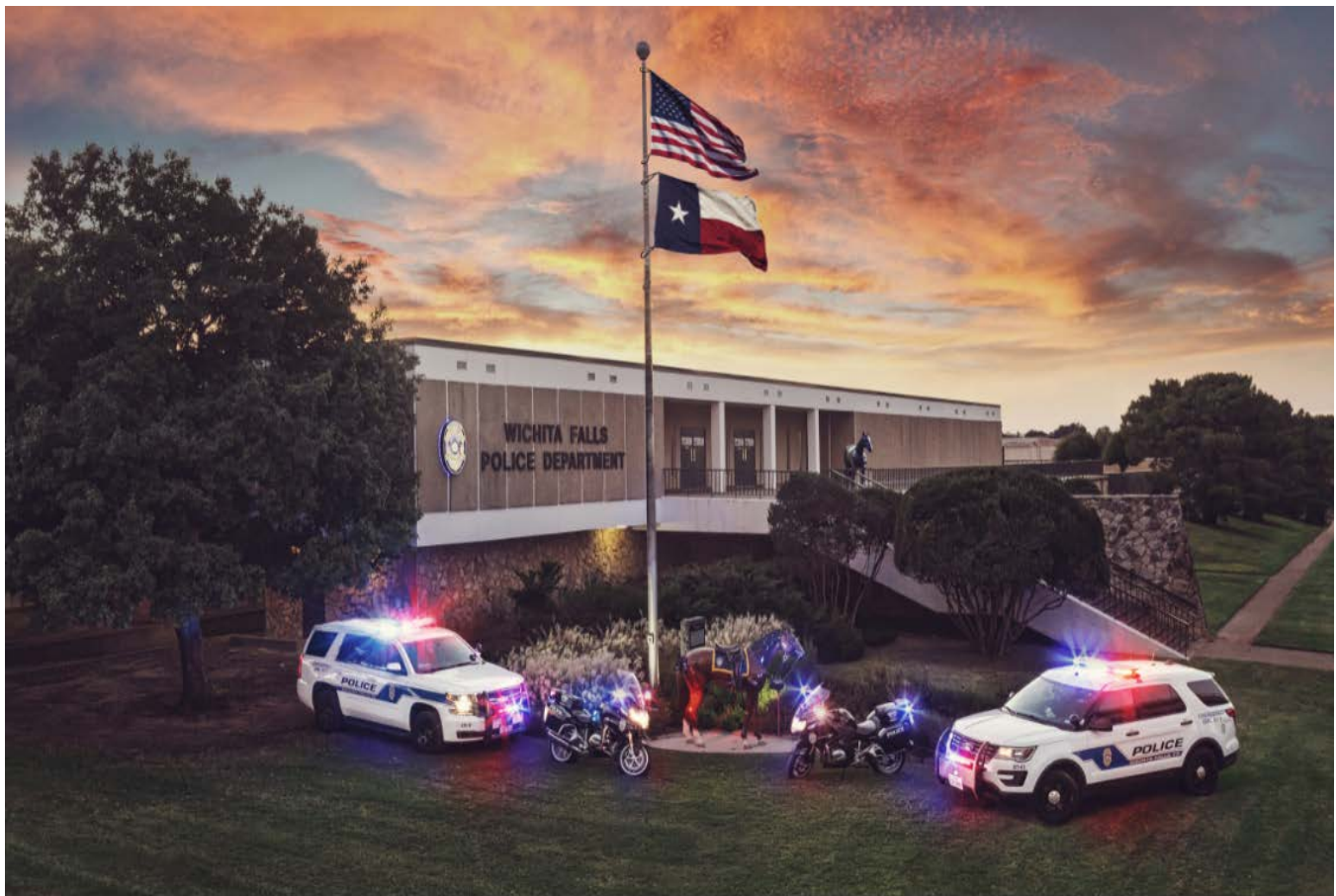
WFPD Headquarters - 610 Holliday Street
